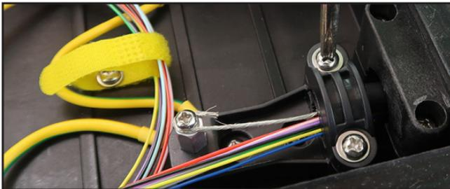
*Figure 1-12: Secure the upper press clamping*
